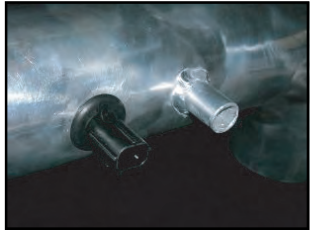
Sensor and Grommet installed in Intake Tube
